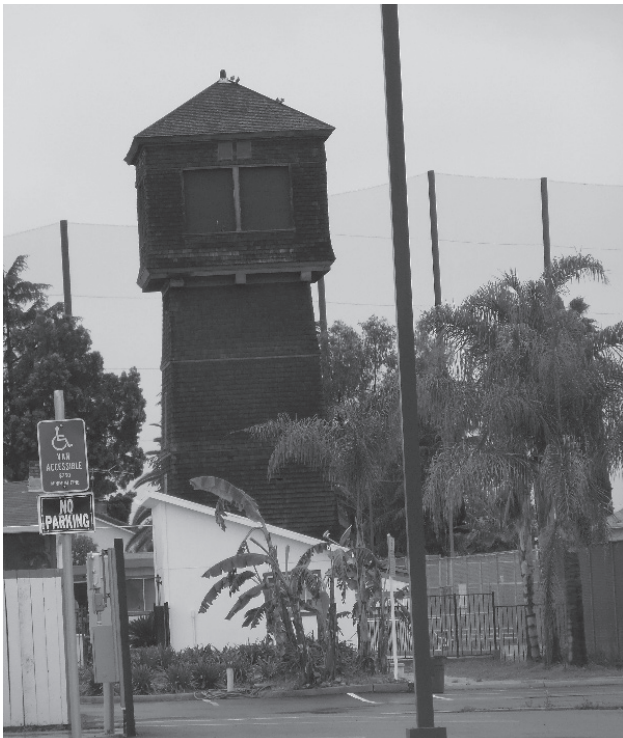
Scenes of modern day near Tully and McLaughlin, San José: a tankhouse/watchtower and a place for San José’s Finest...horses.
