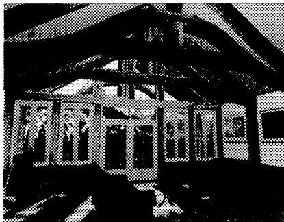
(e) Interior view
