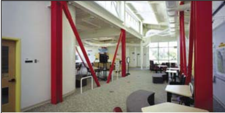
The braces are prominently featured as interior architectural elements.
